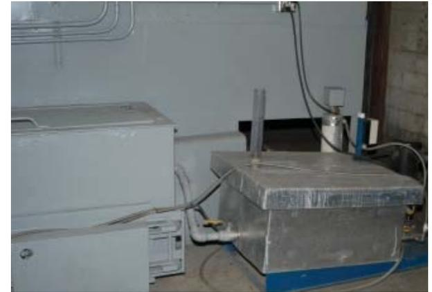
Metcam's new ultrafiltration membrane system installed on Metcam's five-stage pretreatment line continuously removes oil and grease from Stage 1, and ultimately reduces wastewater at Stages 1 and 2. Adding this system and a rinse crossflow system that ties Stages 1 and Stage 2 together reduces wastewater production by more than 76,000 gal./yr. and yields net cost savings for wastewater processing of more than \$29,000/yr.
